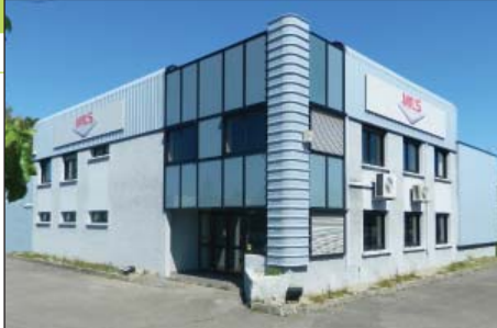
Vacuum pumps site
