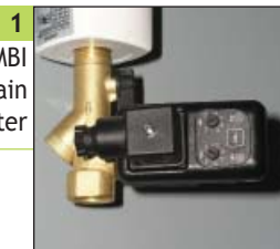
2 BEKO12 electronic drain fitted on the filter
